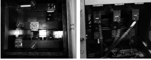
(a) 母线布置 (b) 下柜布置
