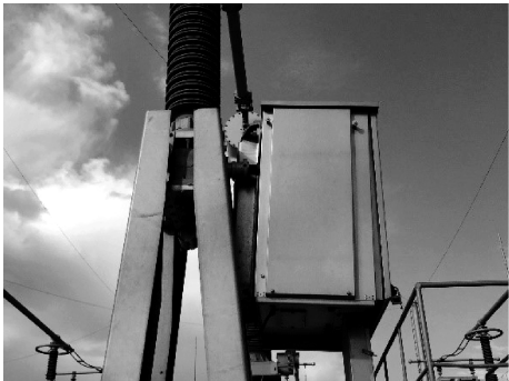
图 1 断路器故障相开关机构箱 Fig. 1 Switch box of fault phase of circuit breaker
